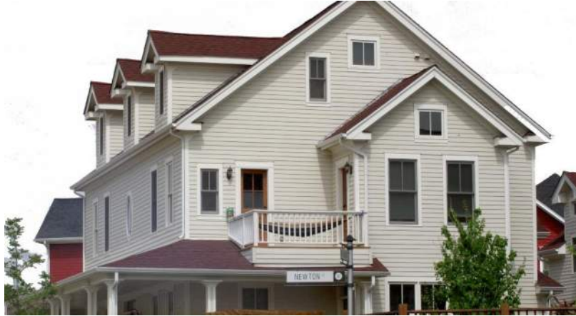
Figure 12-4-2-53 Roof Eaves on Residential Single-Family
