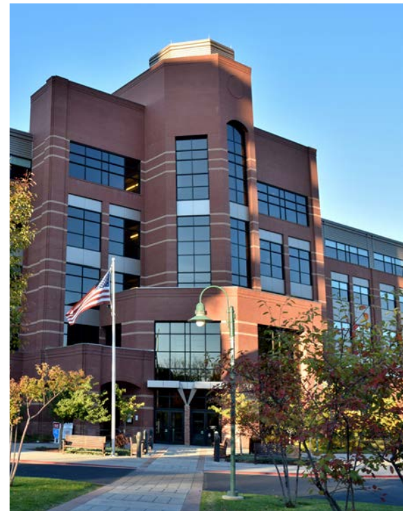
Larimer County Building. Photo: Alisha Jeffers
