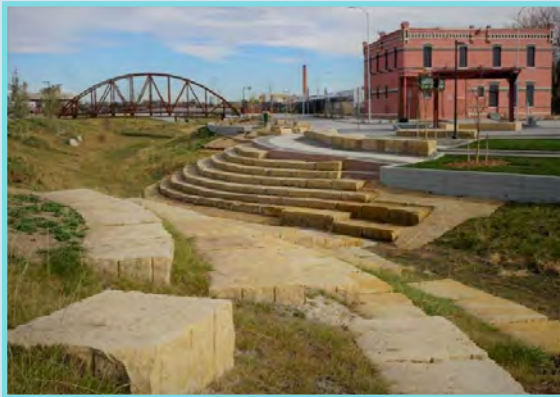
39th Avenue Greenway Project - Denver
